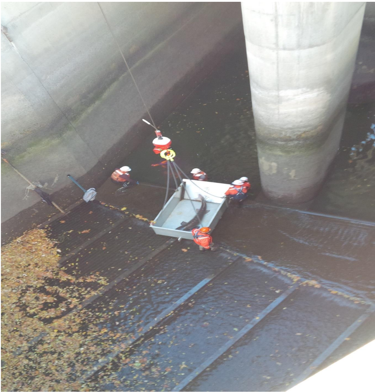
Removing of of 6 large sturgeon from south entrance pool during fishway dewatering.
