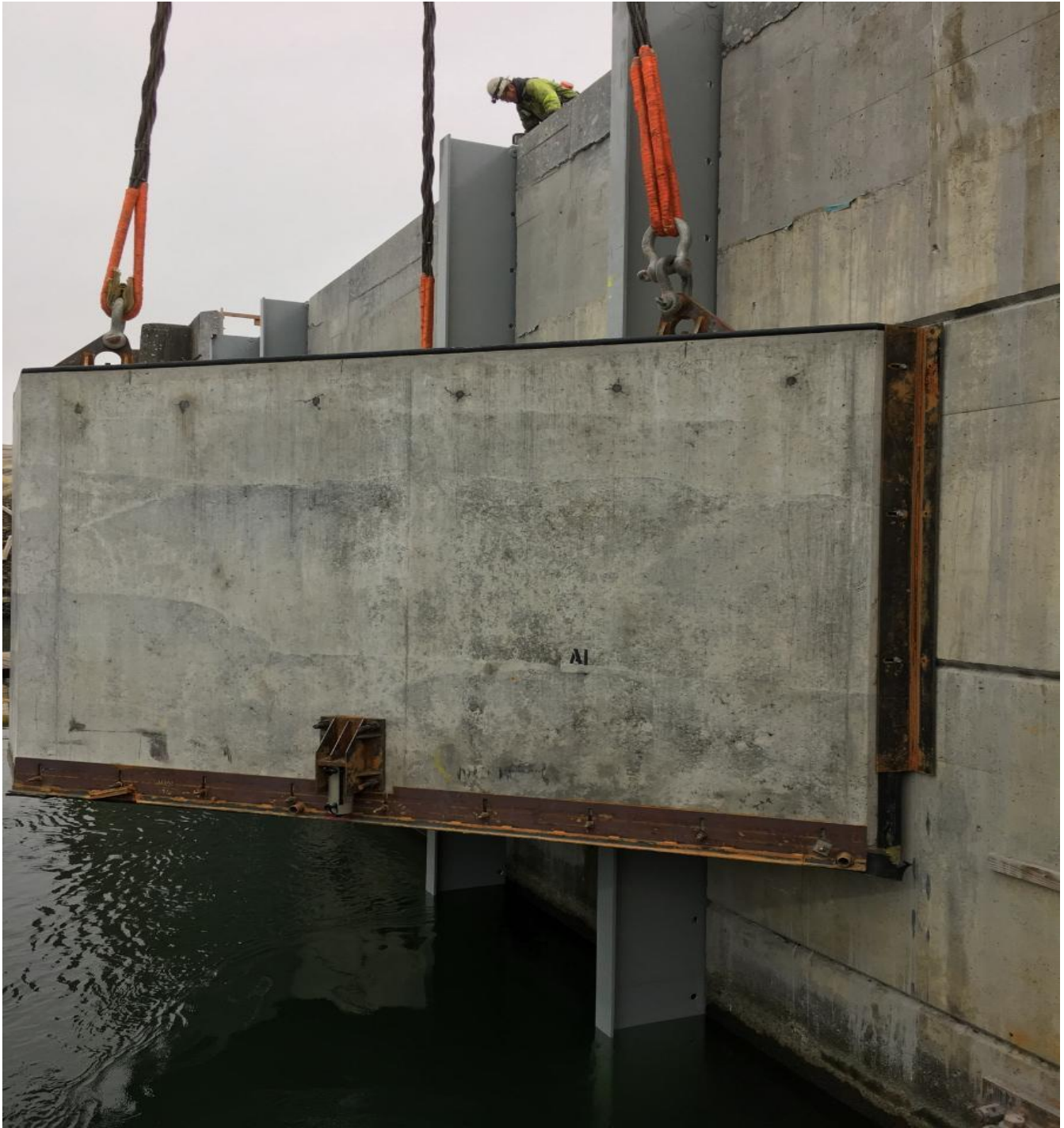
Stacking AWS blocks in forebay
